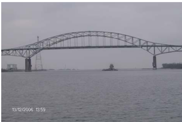
Bridge survey site on Gulf Outlet Canal
