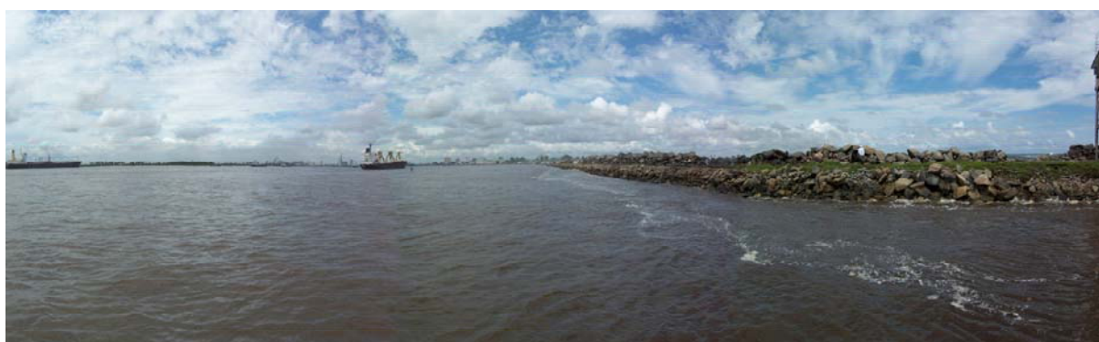
Channel entrance to Lagos Harbour showing LRK station tower on far right.
